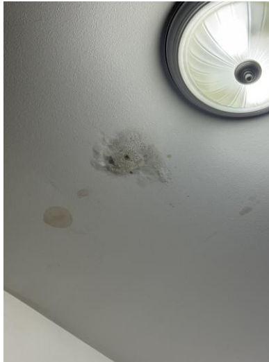
The closet ceiling : the first thing anyone actually saw.
